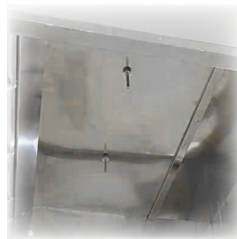
*D-143 Heat Detector in kitchen's hood
